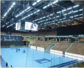
The main hall sound system is built from Bose RoomMatch cabinets, in 10 clusters, driven by PowerMatch amplifiers. Audio and control signals are distributed to the remote racks from the central media room via CobraNet from a Bose ESP-88 DSP units.
