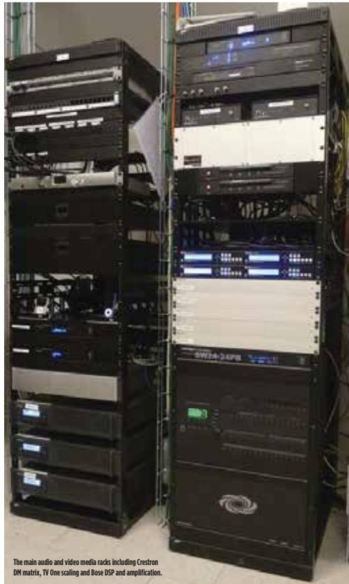
The main audio and video media racks including Crestron DM matrix, TV One scaling and Bose DSP and amplification.
